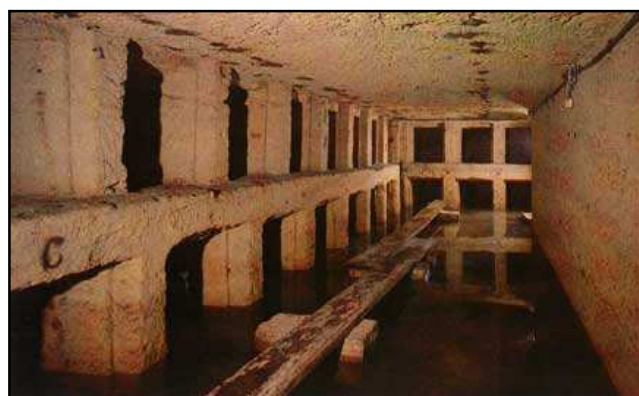
Figure 9. Shows the high levels of water in the first floor of Kom El-Shoqafa catacombs.
