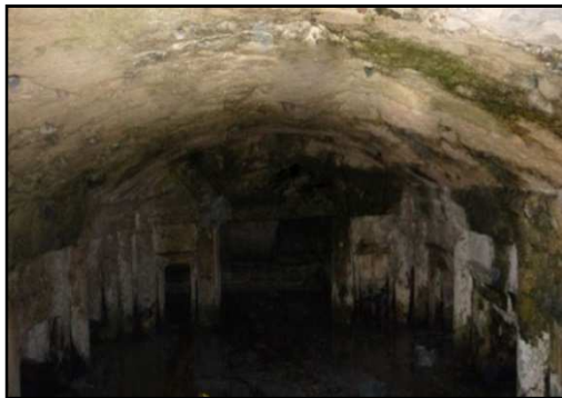
Figure 16. Shows the high growth of algae on the building materials.
