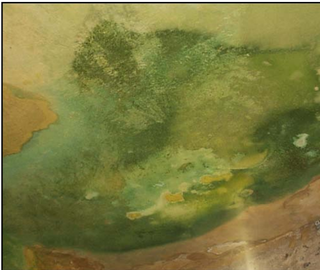
Figure 12. Shows the algae growth on lime stone in Kom El-Shoqafa catacombs.
