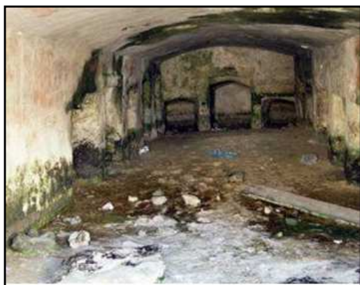
Figure 17. Shows the high levels of water inside the catacombs and also algae growth on the building materials.
