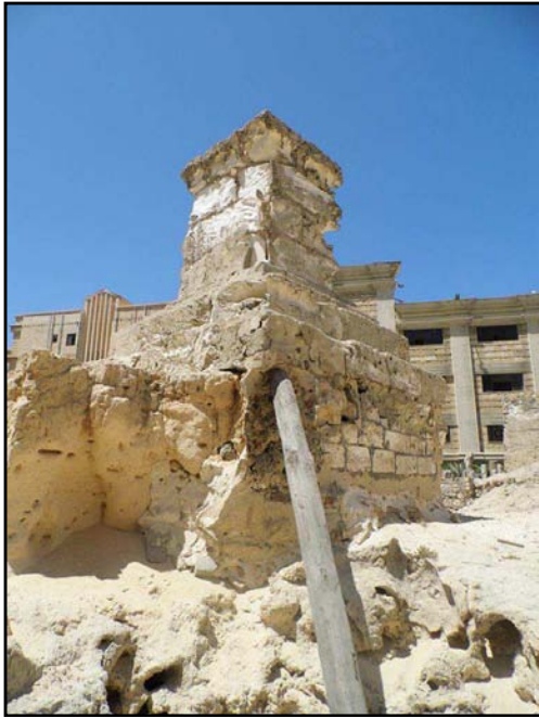
Figure 15. Also shows the wind erosion of the building materials (Fired brick and Lime stone) in the catacombs facades.
