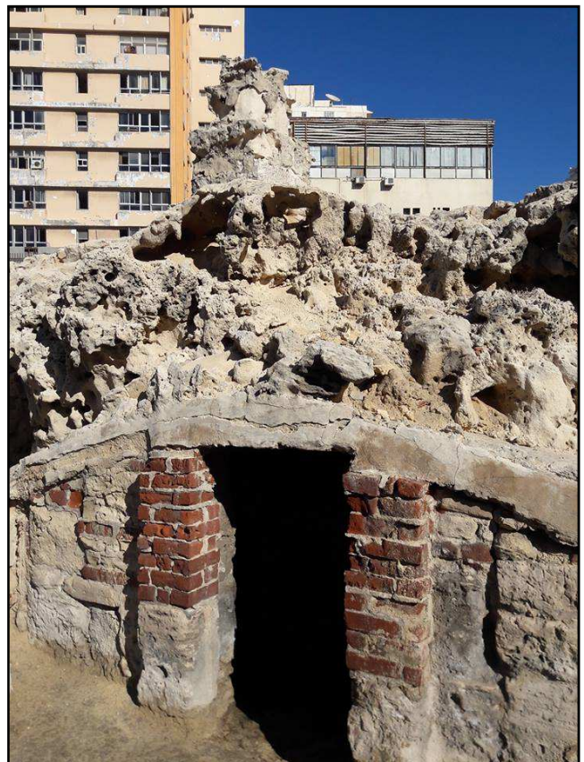
Figure 14. Shows wind erosion of one of the catacombs' facades.
